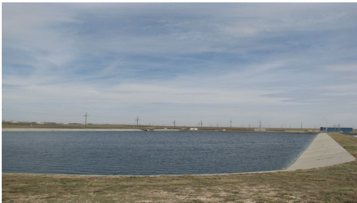
Fig. 8.2. Wastewater Treatment Facility, Facultative Lagoon
