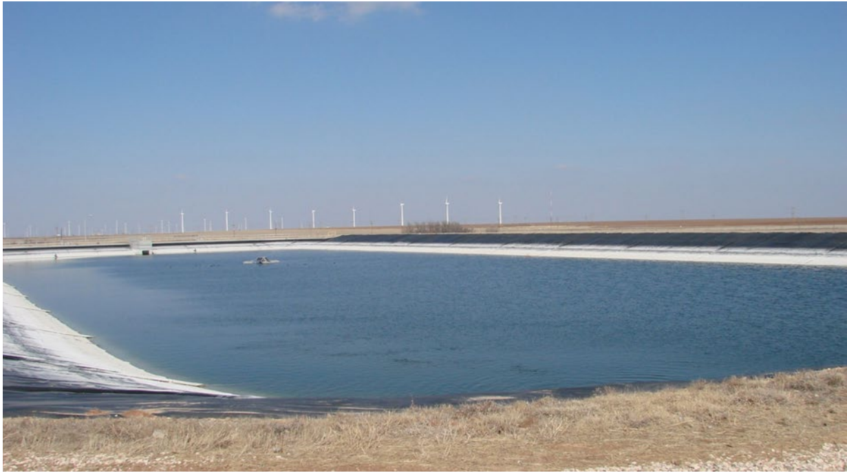
Fig. 8.3. East Wastewater Storage Lagoon
