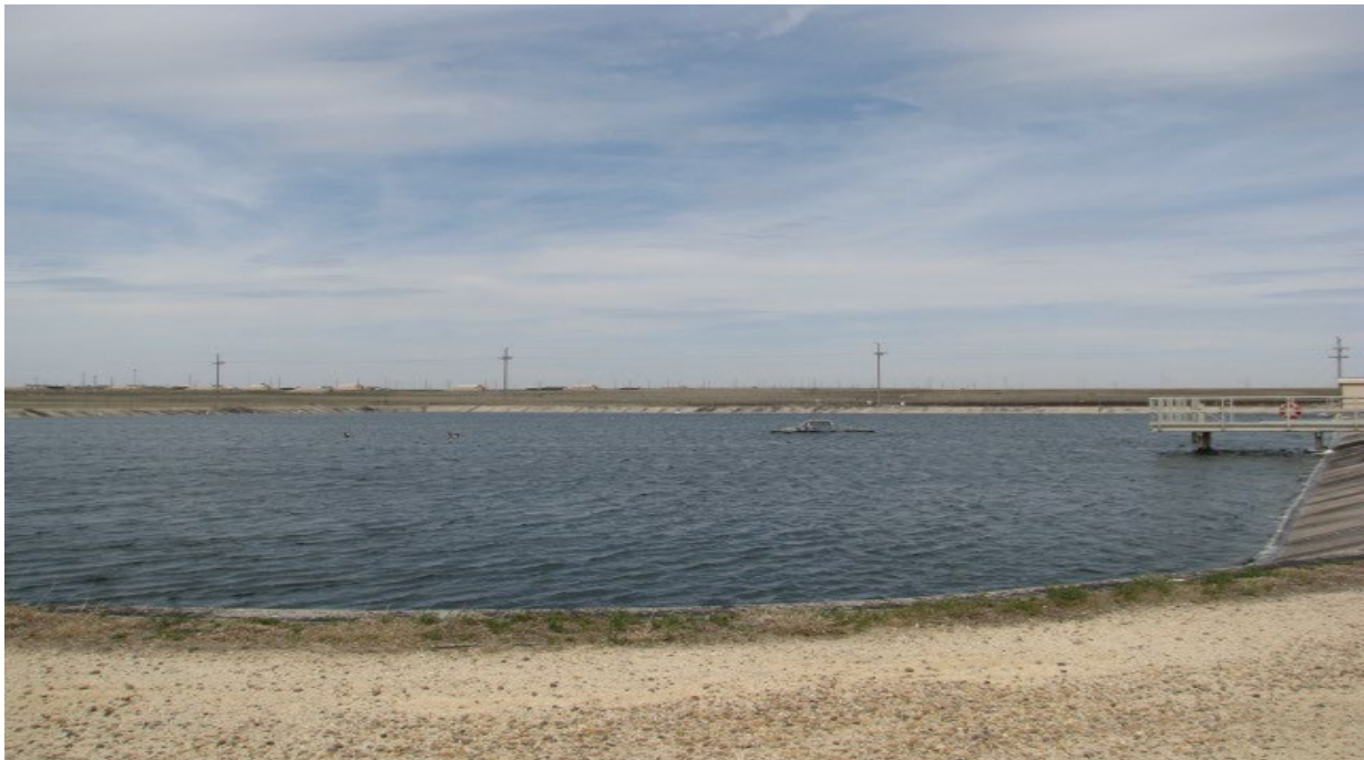
Fig. 8.4. Wastewater Storage Lagoon
