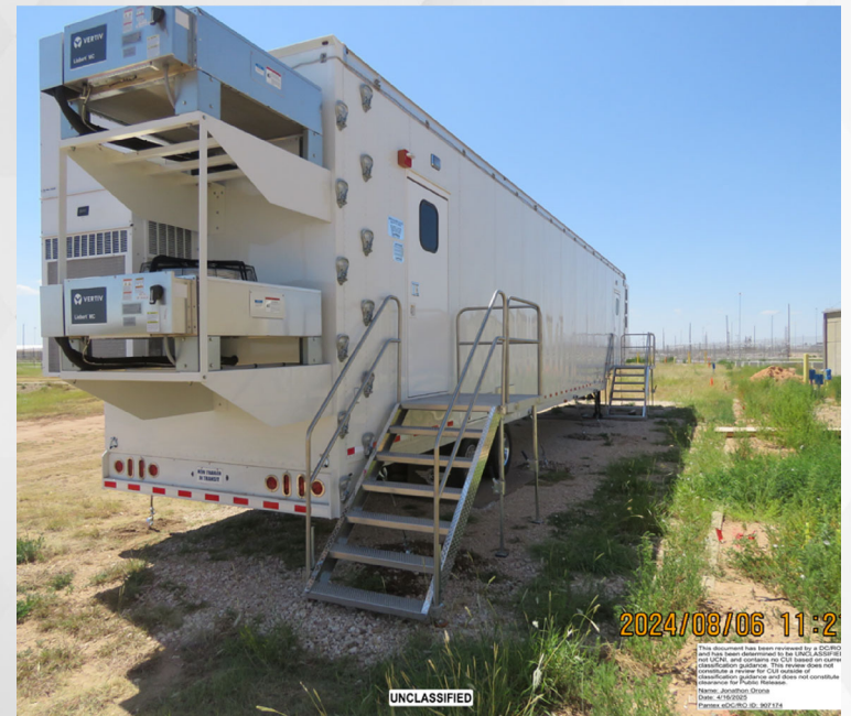
Temporary HVAC trailer to support HVAC replacement
